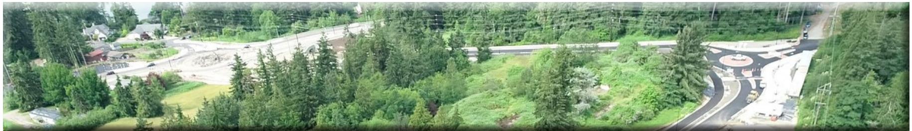
Looking Southwest - Sunrise Ridge Avenue NE, Johnson Parkway, & WA-305
