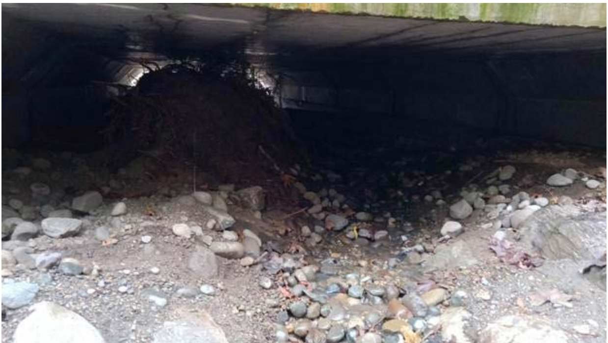
Fig. 4. Material in stream 1 culvert.
