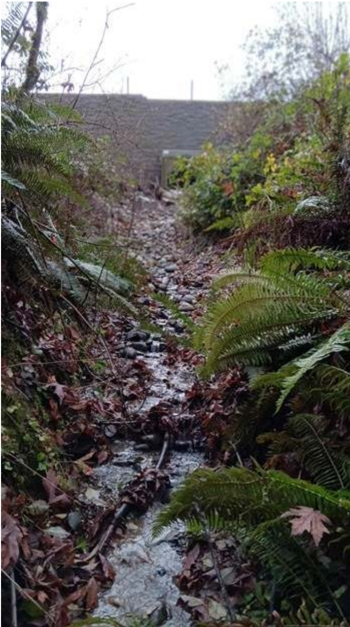
Fig. 2 Looking upstream to where stream 1 passes through a culvert.
