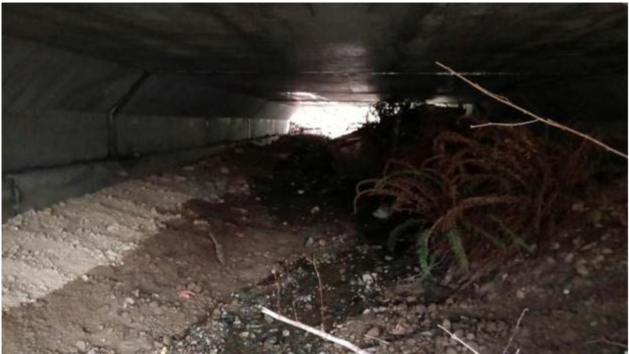
Fig. 3. Material in stream 1 culvert.
