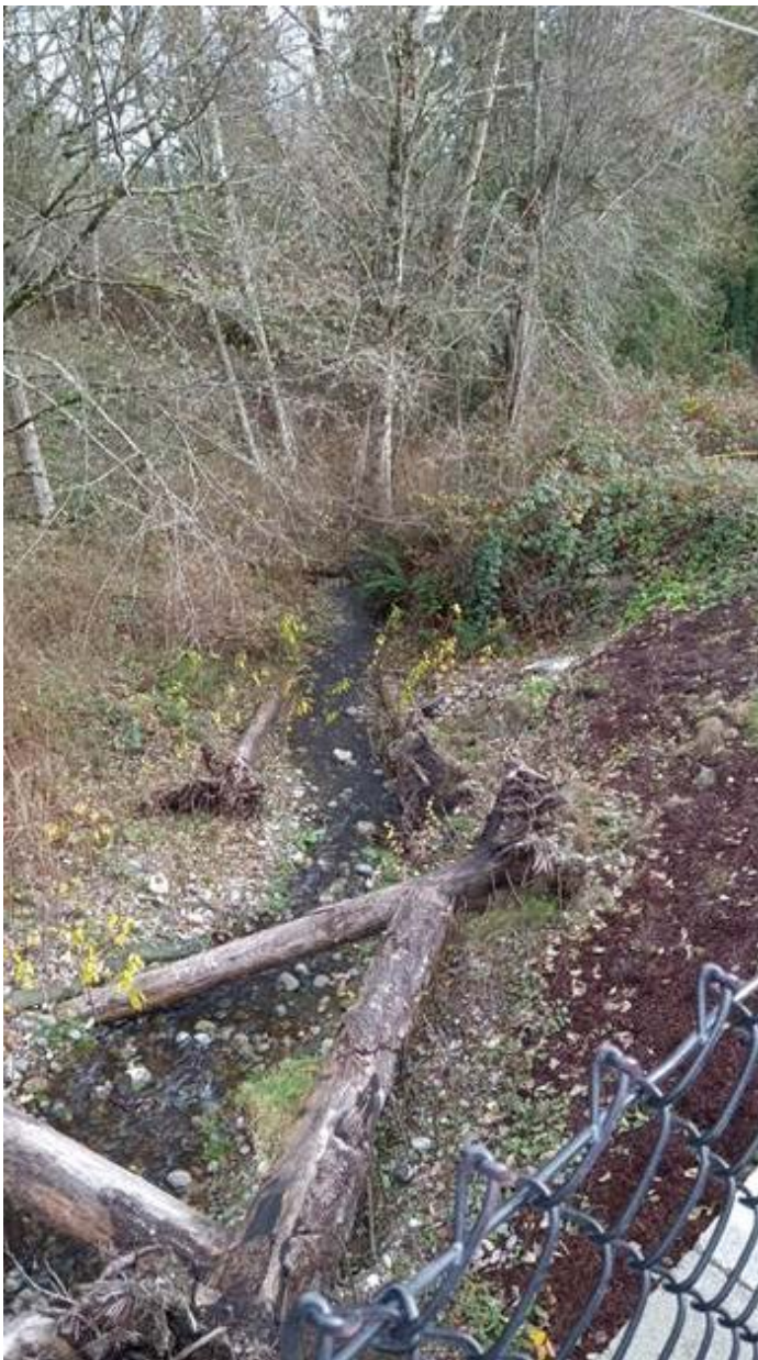
Fig. 1. Work on Bjorgen Creek.
