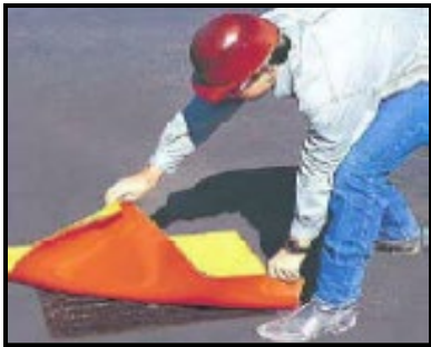
B. Seal storm drains using a plug or rubber mat
