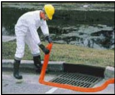
A. Create a barrier around storm drains using spill berms, sandbags, or plastic sheeting
