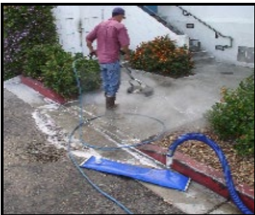
C. Collect washwater using a vacuum boom or containment pad.
